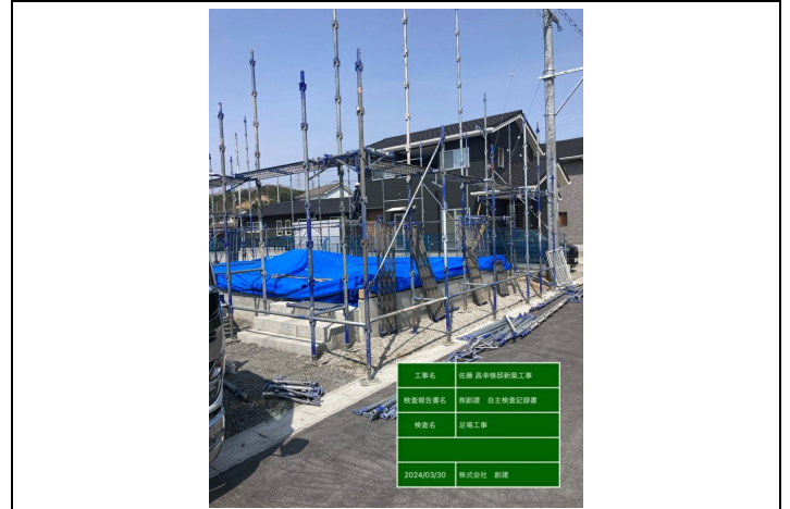
☑組立施工中①
