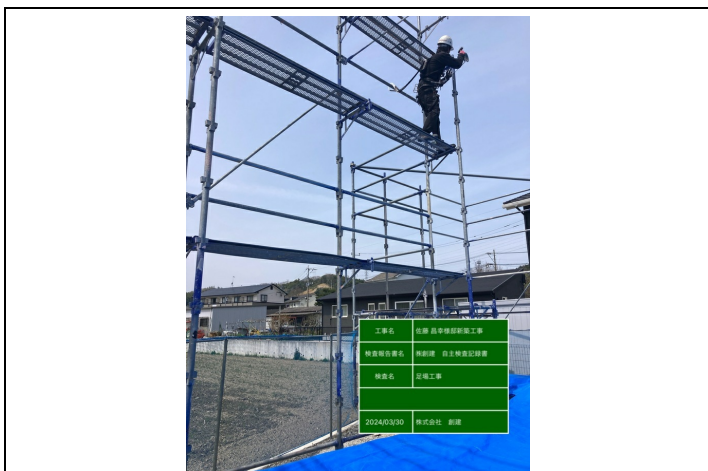
☑組立施工中①
