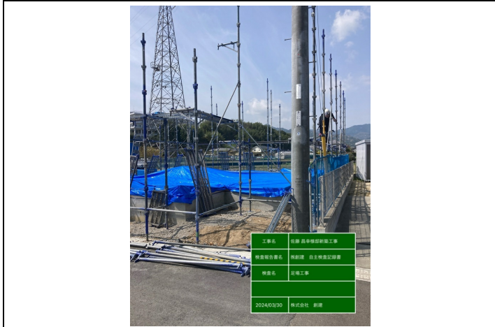
☑組立施工中①
